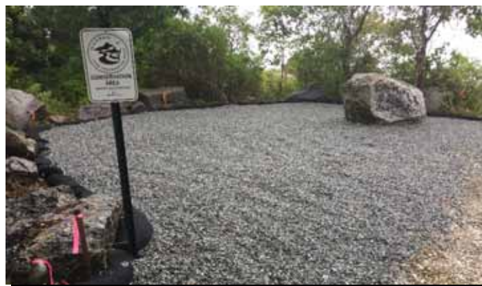
Completed parking spaces – Toweset Landing
